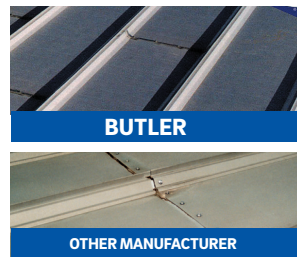
Above Top: Butler staggers panel splices to avoid the four-corner condition—another design feature to assure weathertightness and longer roof life. Above Bottom: Most manufacturers locate panel splices at exactly the same position across the roof. This four-corner condition is very difficult to seal and keep weathertight.
