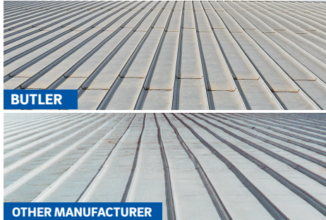
Above Top: Butler's factory punching assures straight panel alignment. Above Bottom: Without factory punching, these misaligned panels bind on clips, strain seams and compromise weathertightness.
