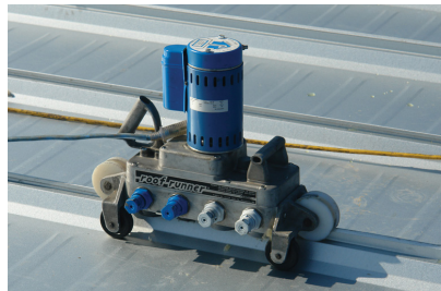
Butler's exclusive Roof Runner® completes the industry's only field-formed 360-degree Pittsburgh double-lock seam.
